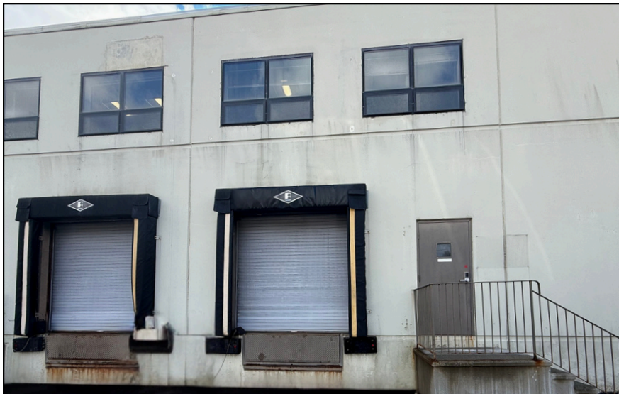
TWO LOADING DOCKS EACH WITH A LEVELER
