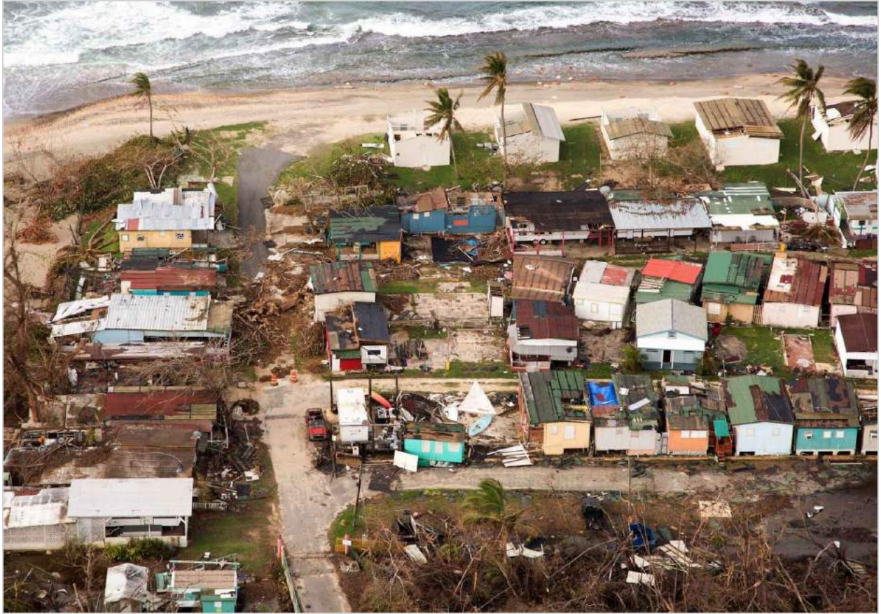
Puerto Rico suffered massive damage from Hurricane Maria in 2017.
