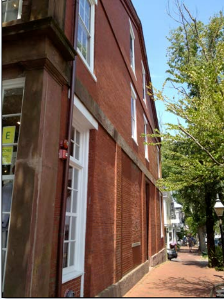
Federal Street View
