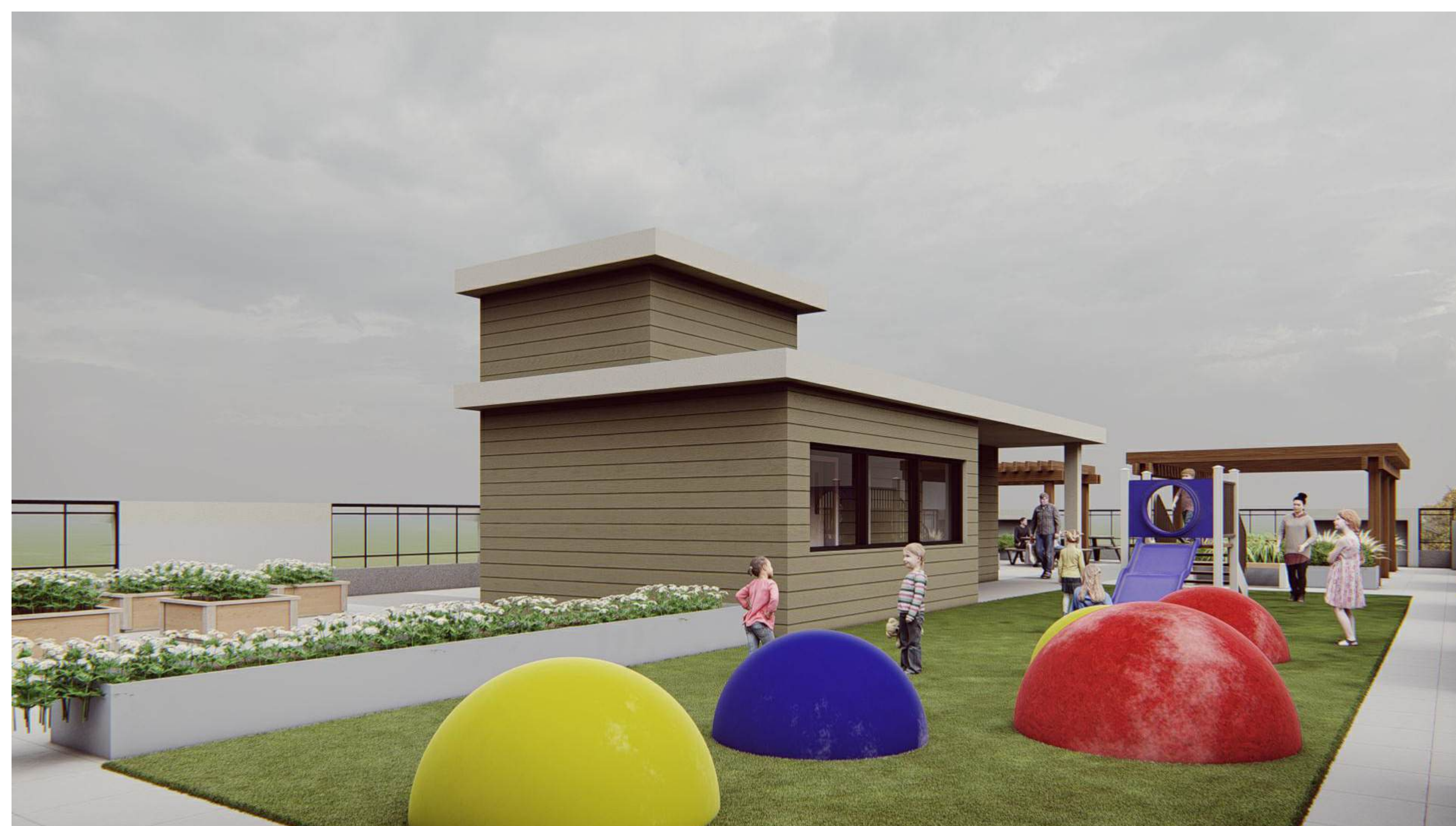
VIEW AT ROOF DECK
