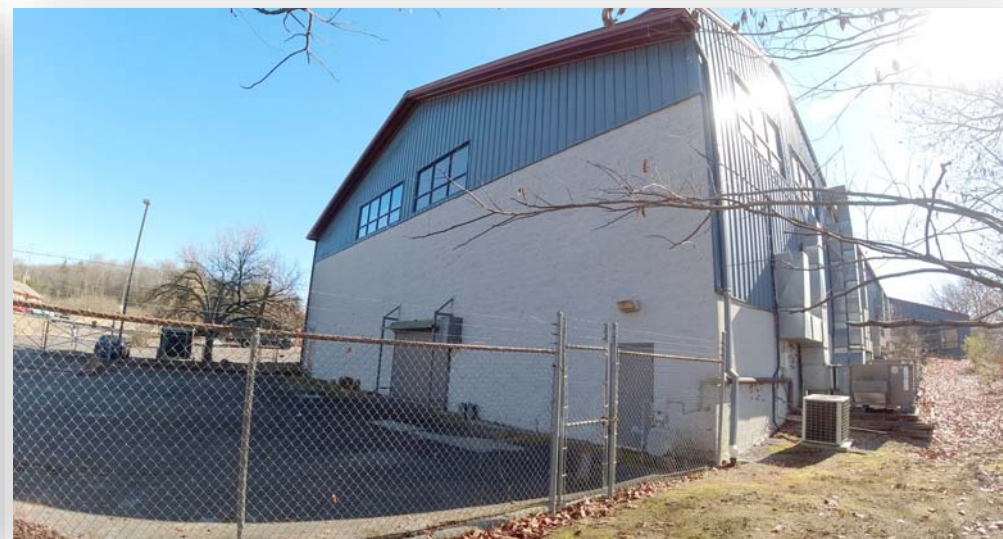
North End of Building Lower Level Entrance
