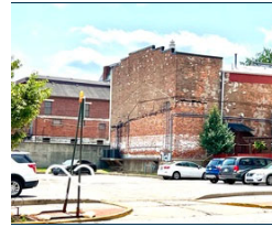
Rear of the building.
