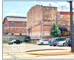
Rear of the building.
