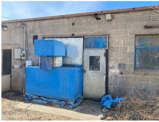
Outside Back of Bldg, Paint Equipment
