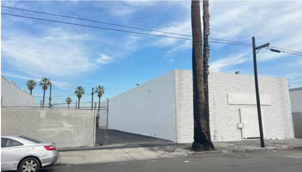
Front of Building
