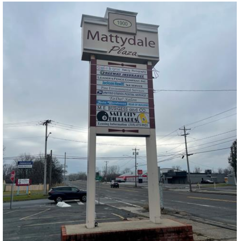
Pylon Sign – Facing Brewerton Road
