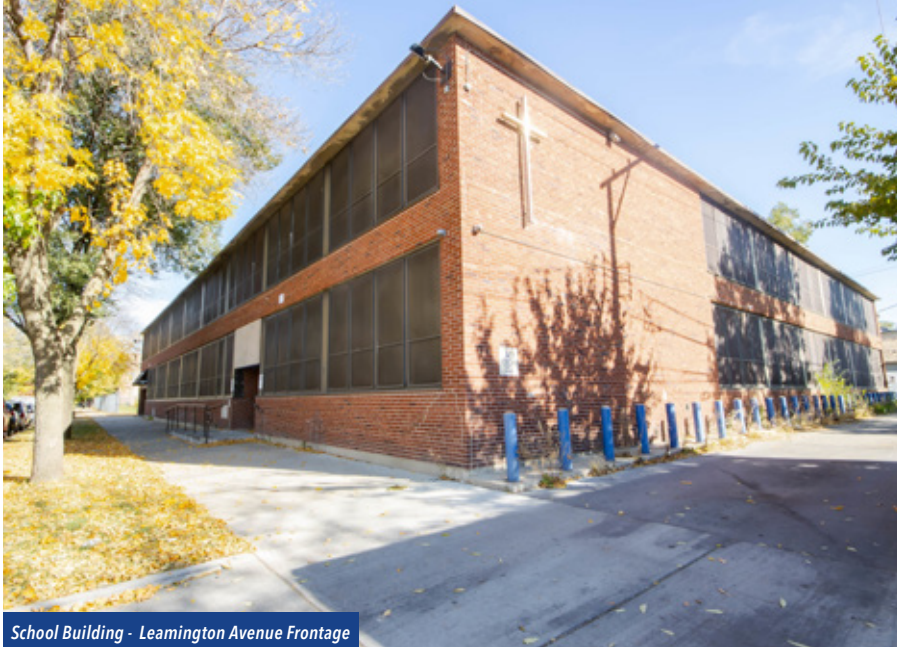
School Building - Leamington Avenue Frontage
