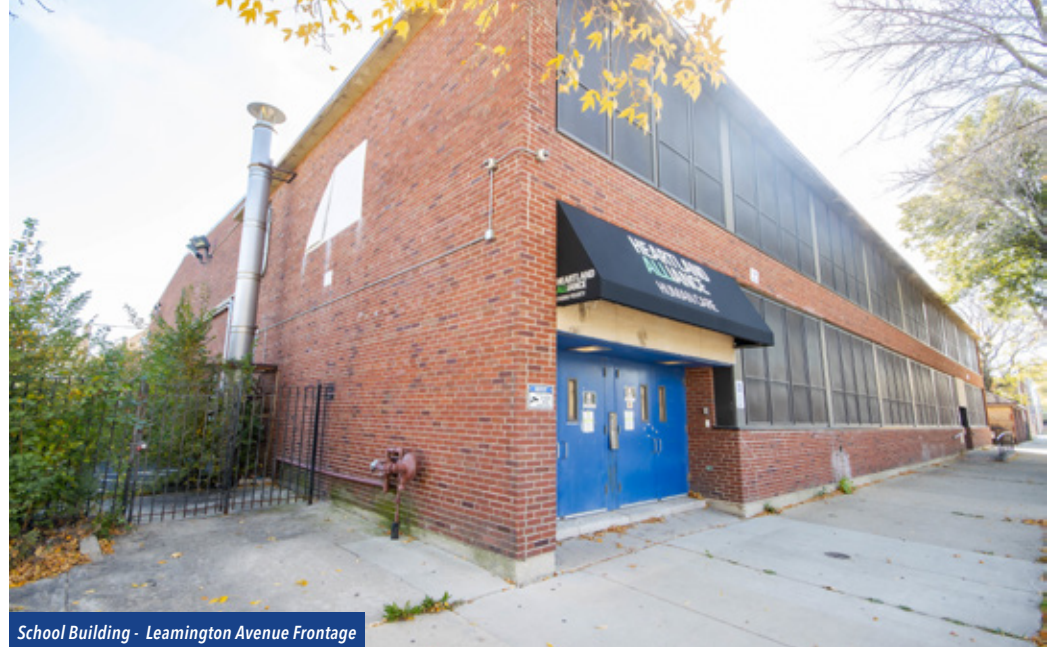
School Building - Leamington Avenue Frontage
