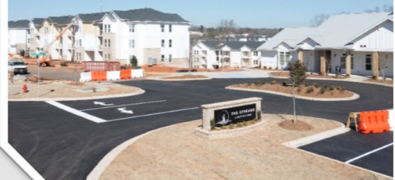
The Streams at Battery Park 264 Units—Completed
