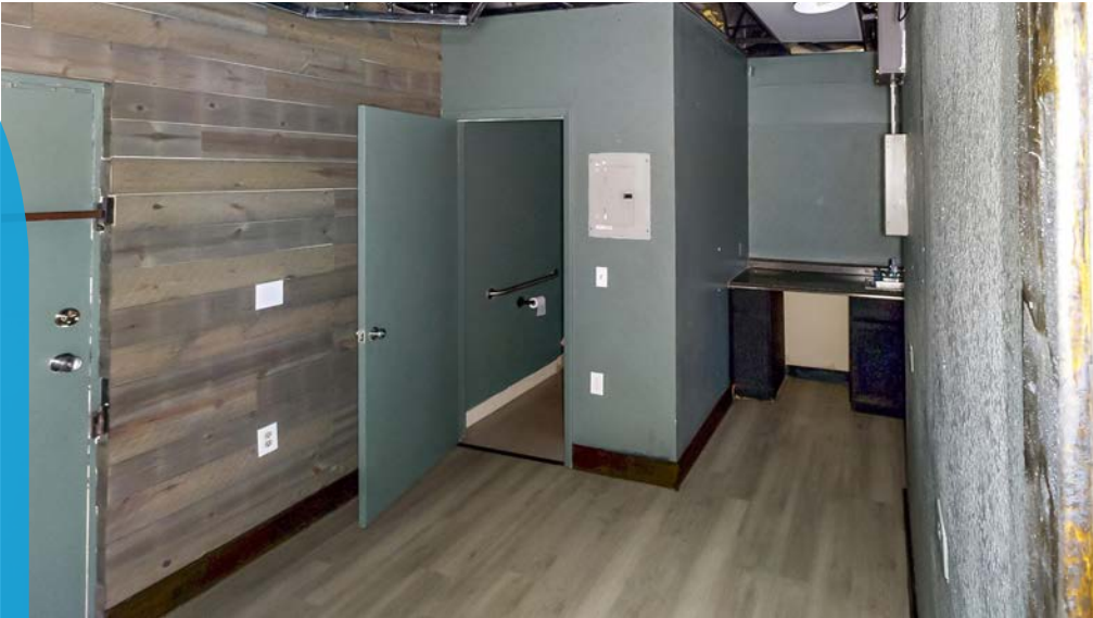
back area | restroom
