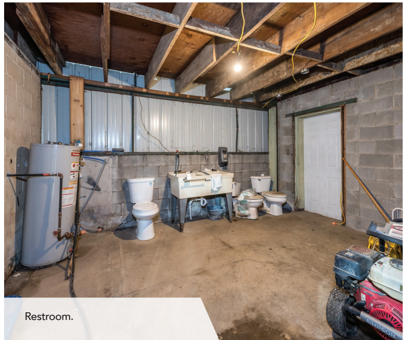
Open Industrial Space.
