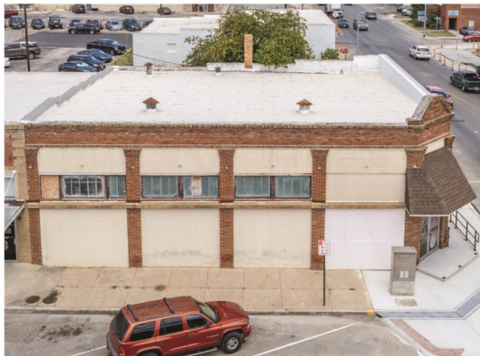
Existing conditions - West Façade.
