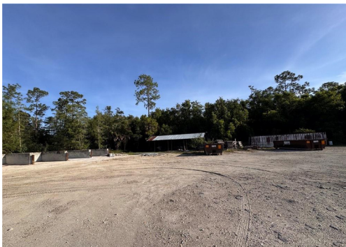
OPEN YARD / SERVICE AREA
