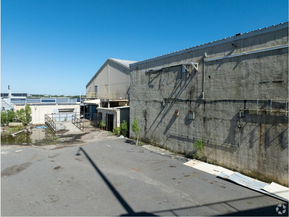
Rear of Buildings
