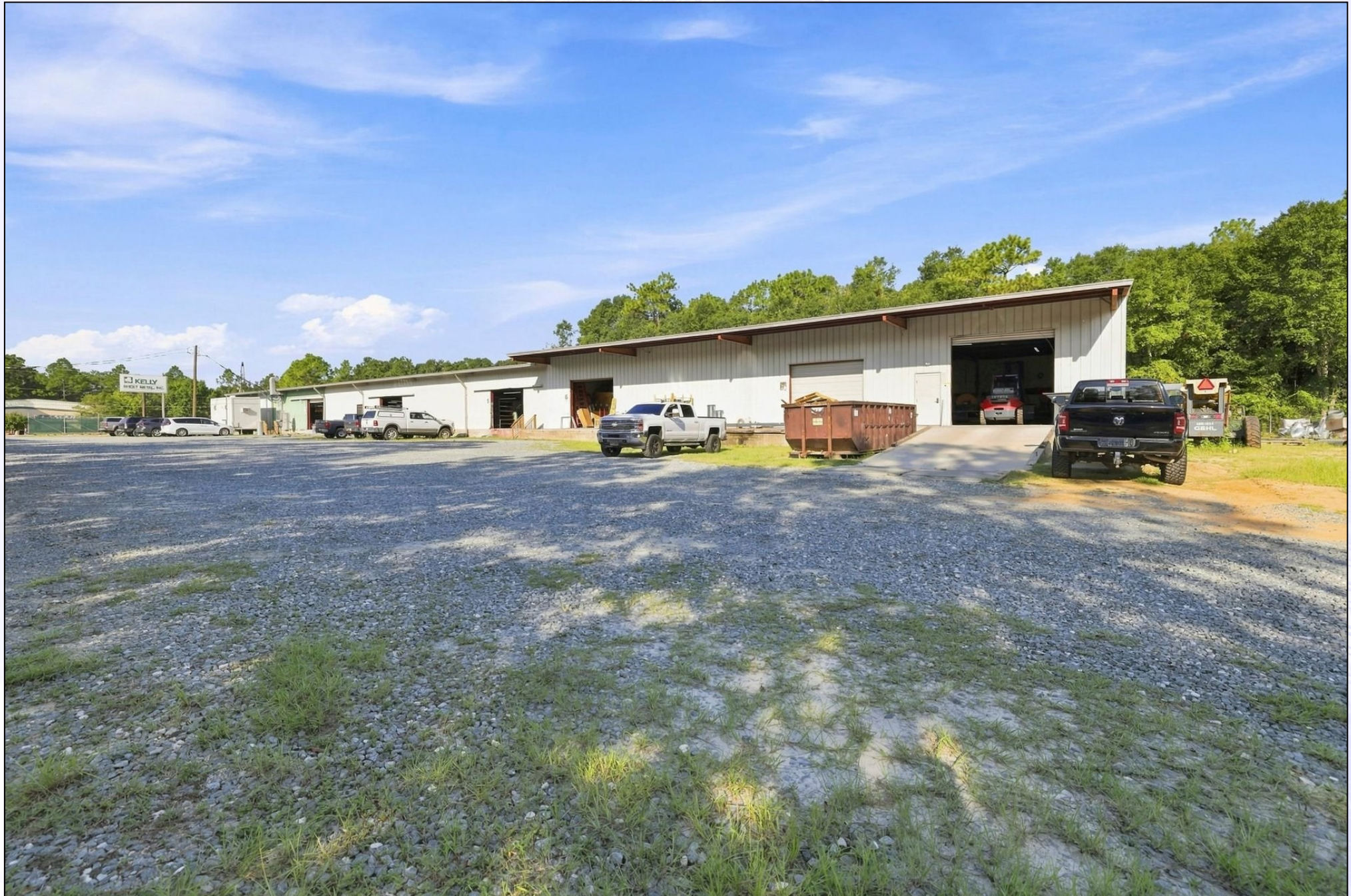
Building Exterior-Side View
