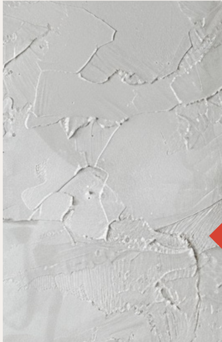
CALIFORNIA STUCCO FINISH FEATURING A HAND TEXTURED SURFACE FOR A CLASSIC LOOK
