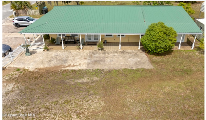
REAR IMPROVEMENTS AND COVERED WORK/STORAGE AREA
