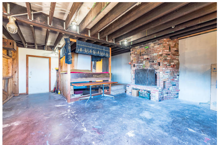
Large living quarters equipped with custom brick fireplace.
