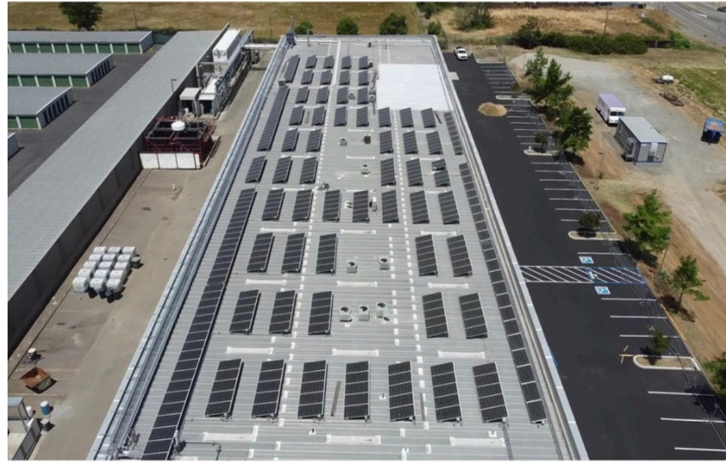
Roof Mounted Photovoltaic System
