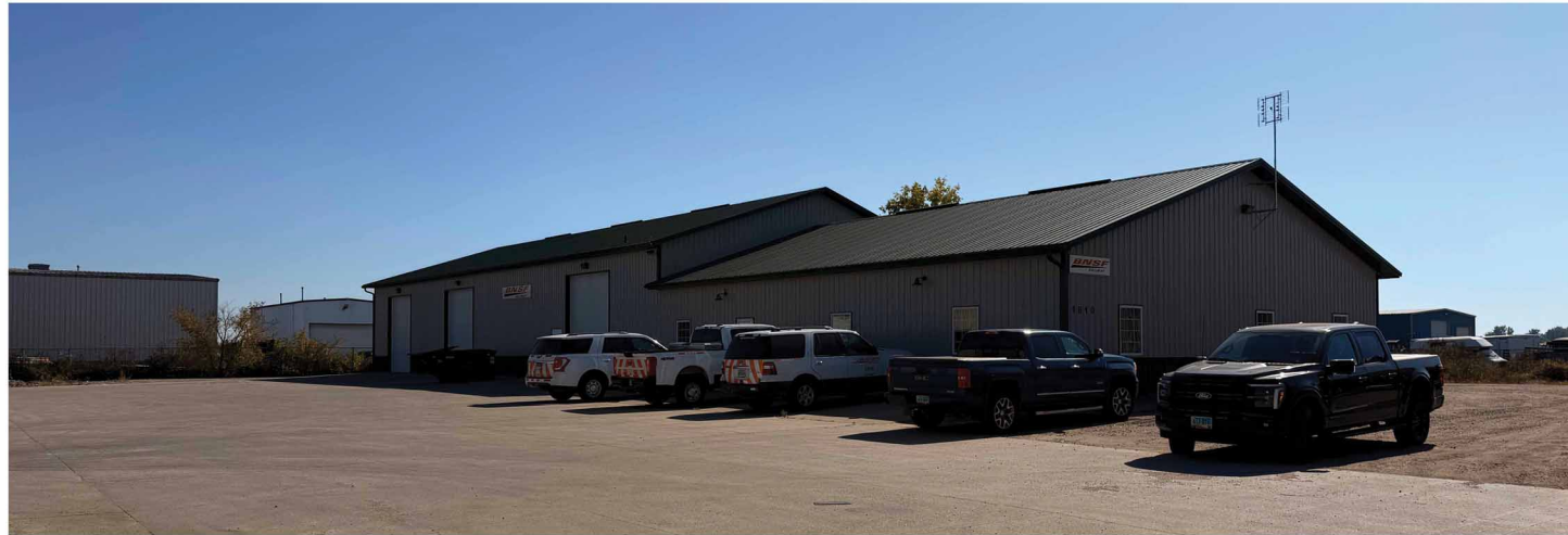
Building 4: 200 amp, three phase 120/209, one meter that also feeds Building 2.
