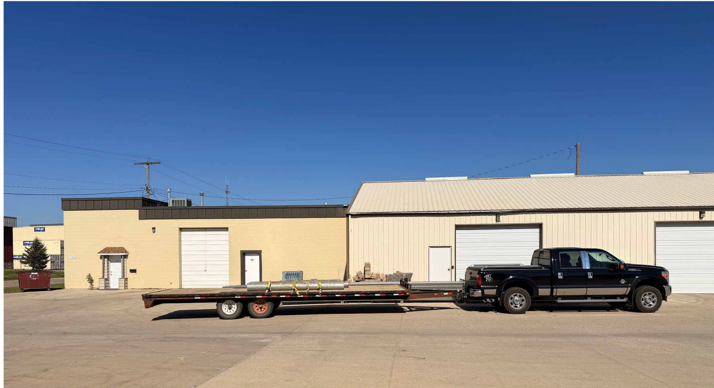
Building 1: 200 amp, single phase, 120/240
