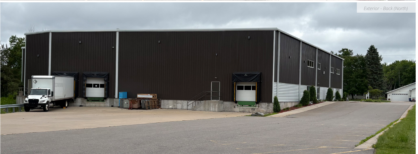
Exterior - Front (South)
