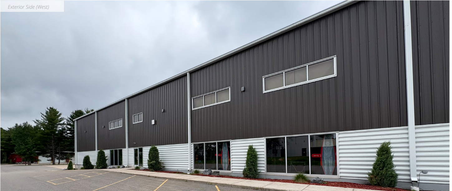
Exterior - Back (North)
