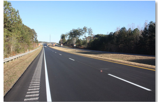
Above: U.S. Hwy 278 East. Property to the Right.
