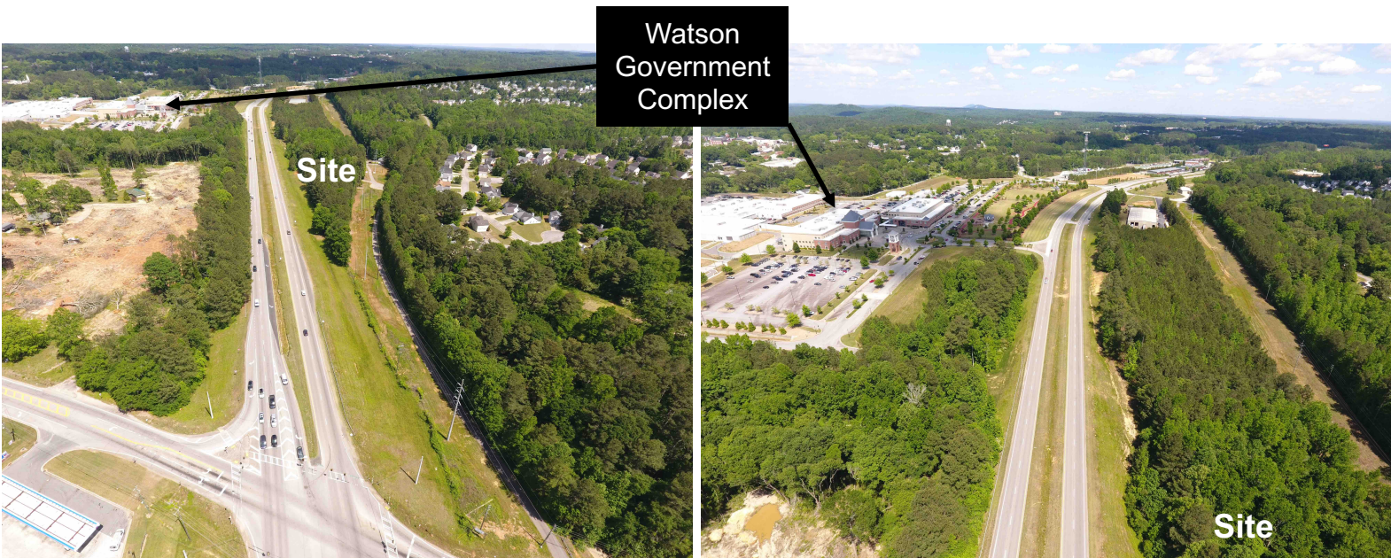
Aerial View Looking East from Hwy 120/Hwy 278 Intersection
