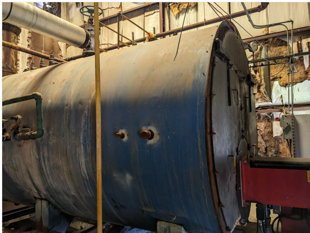
Plant 3 Bldg interior
