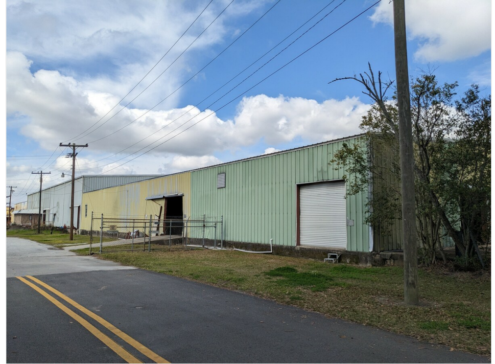
Plant 1 Bldg North
