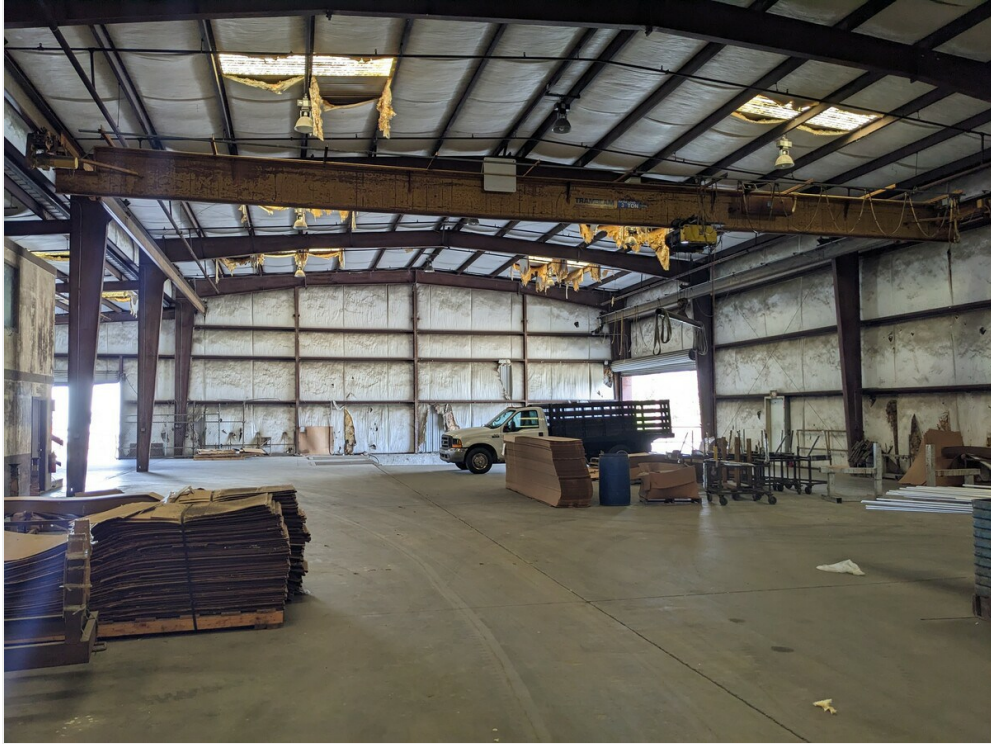
Plant 3 Bldg interior
