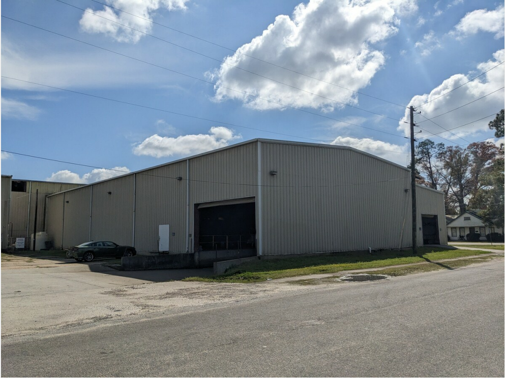
Plant 3 Bldg South
