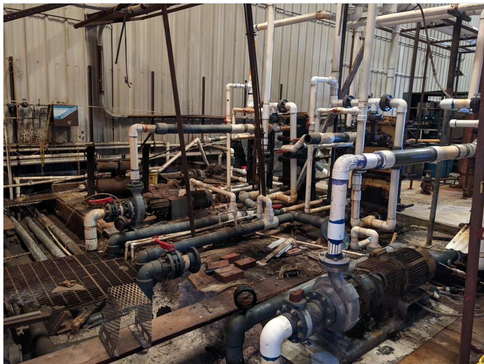
Plant 3 Bldg interior
