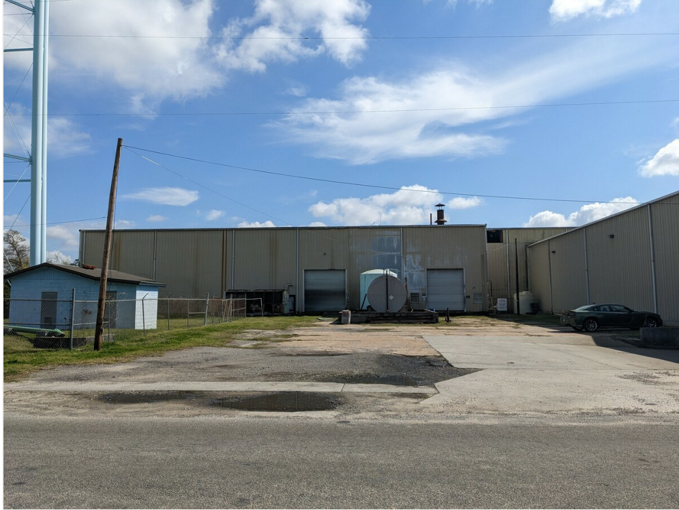
Plant 3 Bldg South
