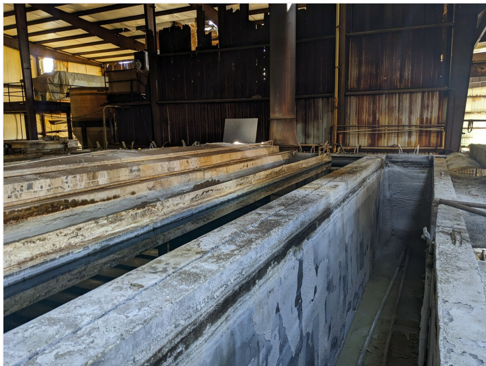
Plant 3 Bldg interior
