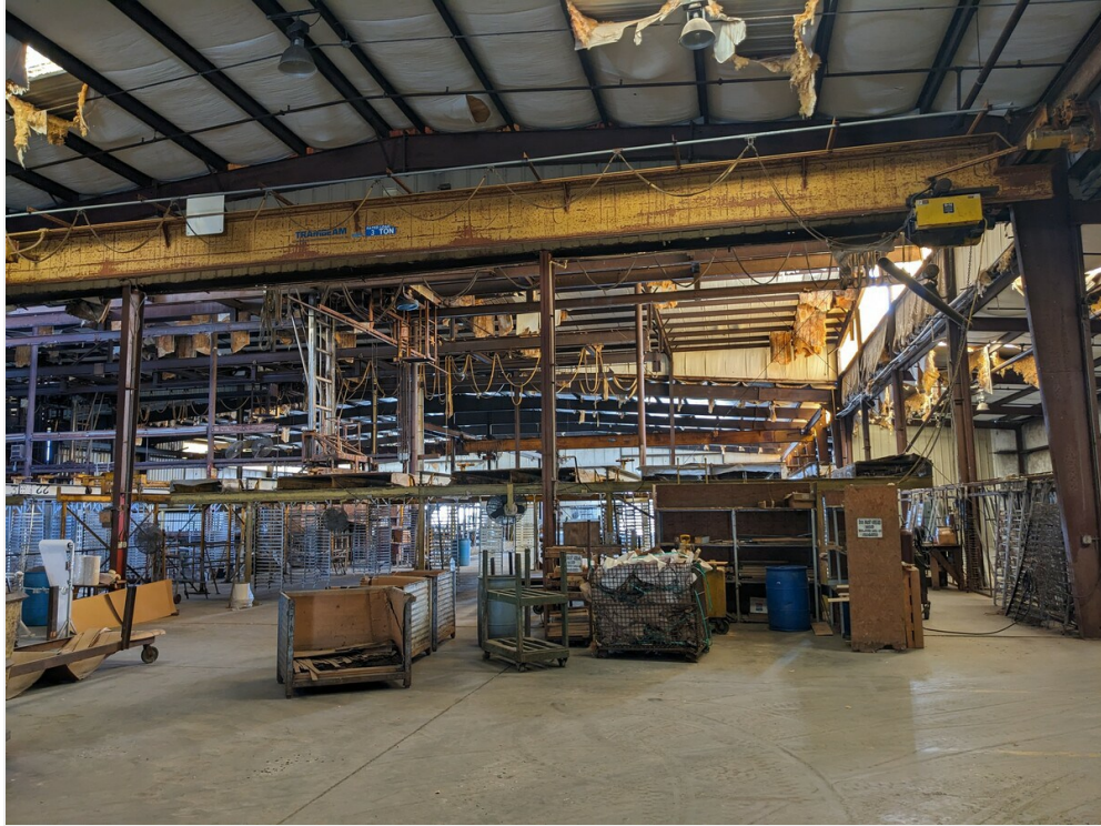
Plant 3 Bldg interior
