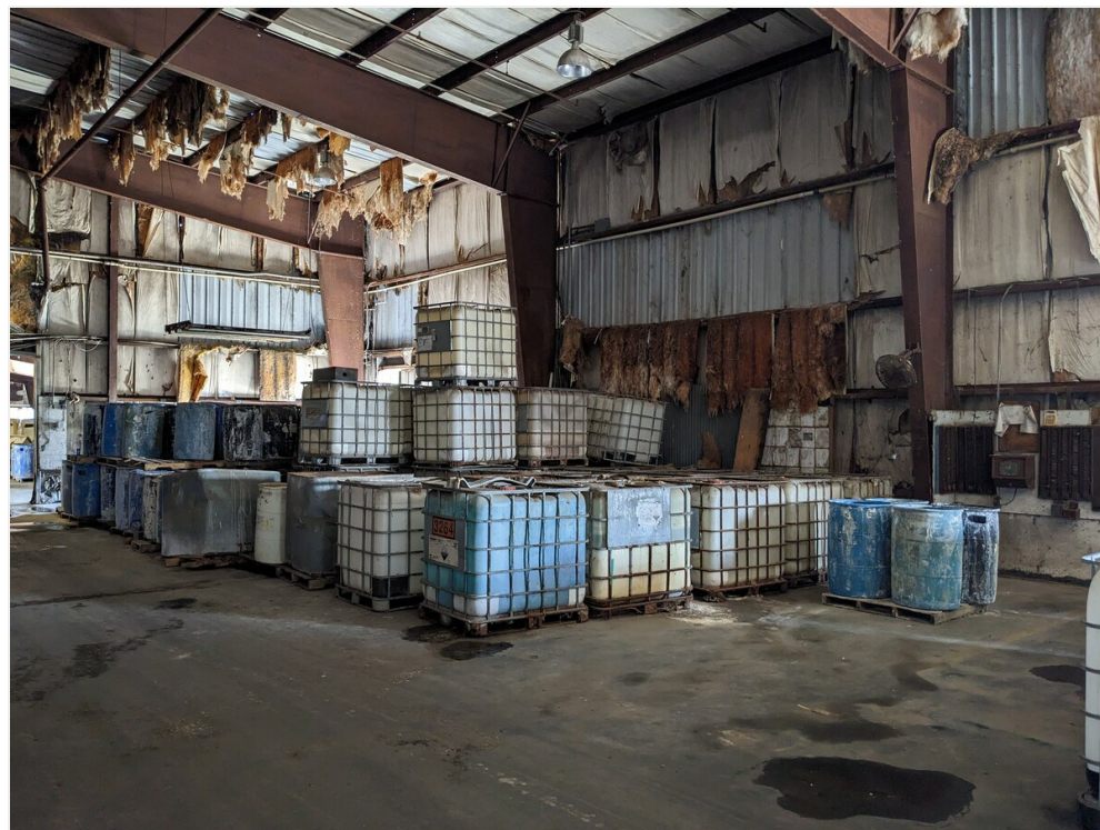
Plant 1 Bldg interior
