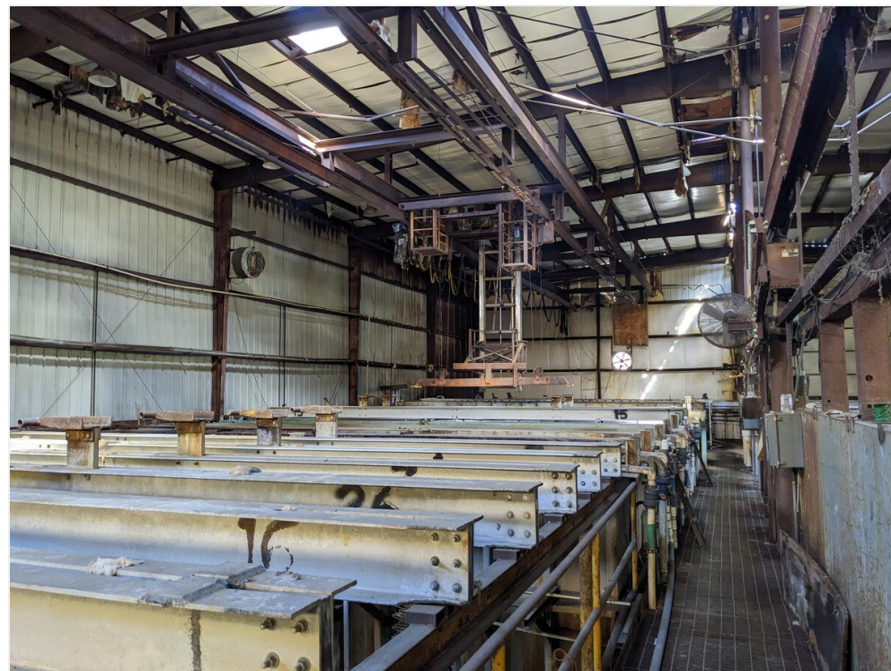
Plant 3 Bldg interior
