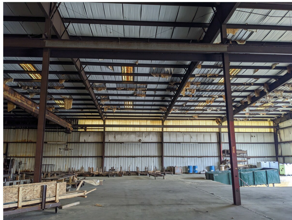
Plant 3 bldg interior
