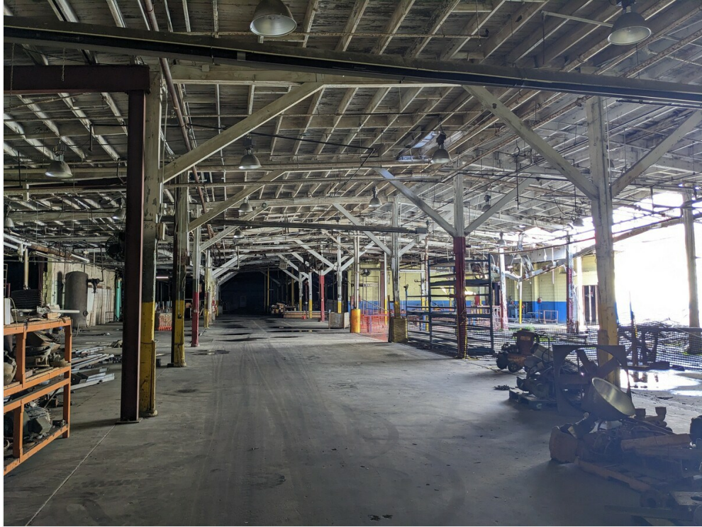
Plant 1 Bldg interior
