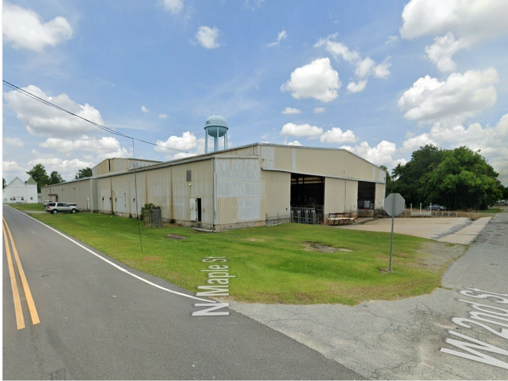
Plant 3 Bldg South
