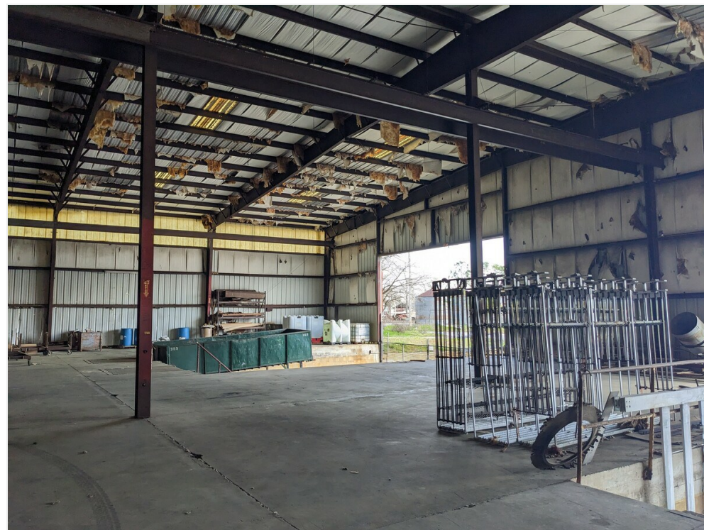
Plant 3 Bldg interior
