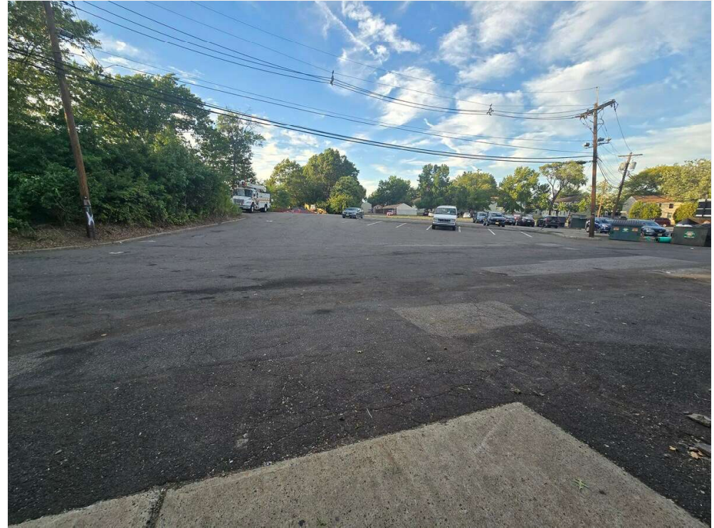
rear parking lot
