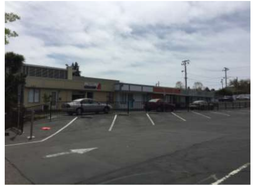
Photo 2: View looking southwest toward site, across neighboring parking lot
