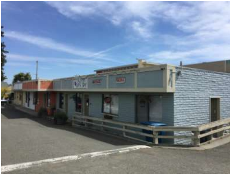
Photo 3: View looking southeast at site building
