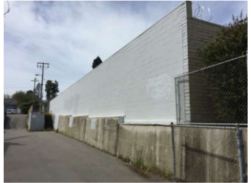
Photo 6: View of rear of site building
