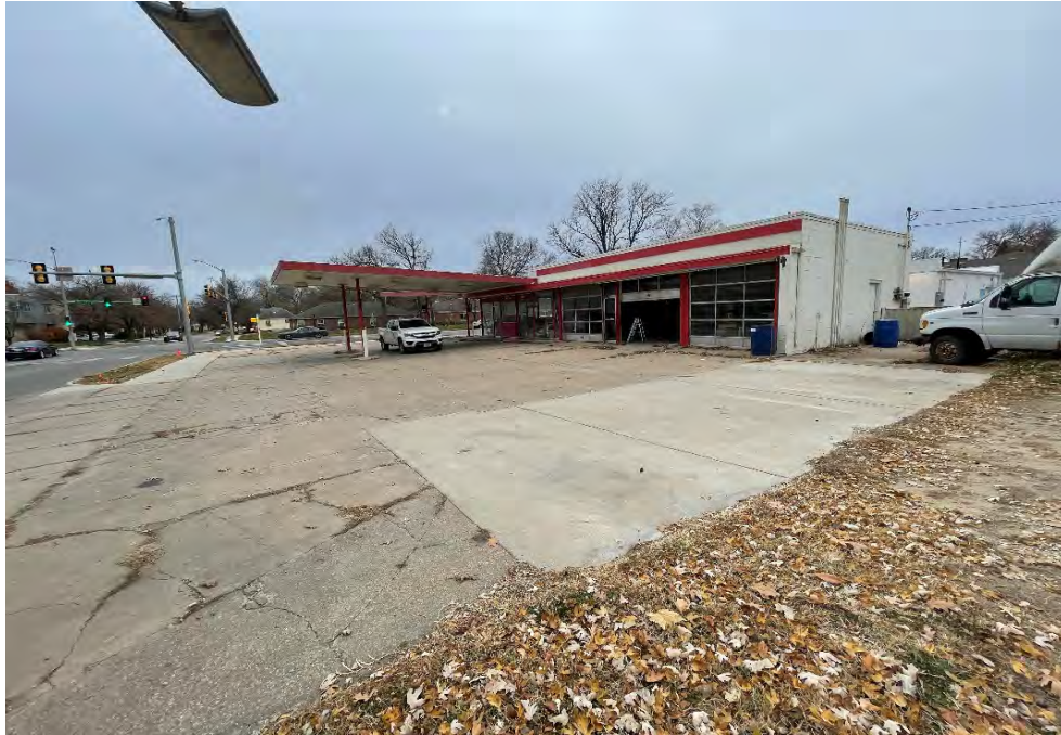
1. View of onsite retail petroleum structure.
