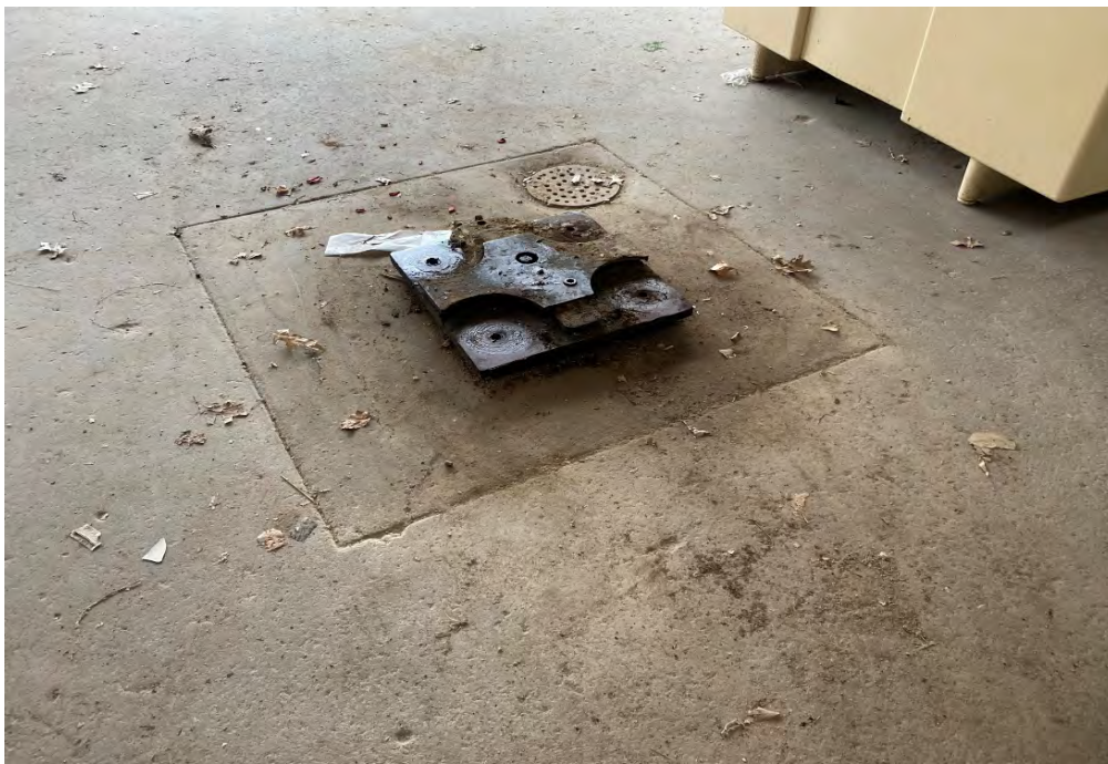
10. Representative view of underground hydraulic lift observed at the site.
