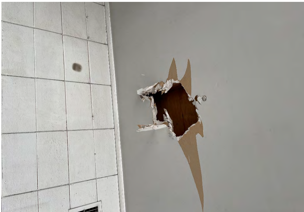
2. View of drywall joint compound (Sample 2-2) containing <1% chrysotile asbestos.
