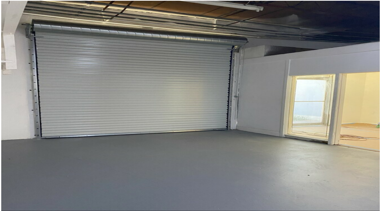
suite 1 warehouse showing new roll up
