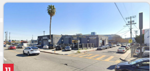
11 100 Apartments 11044 Burbank Blvd
