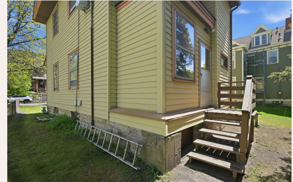
Rear stairs to unit 1
