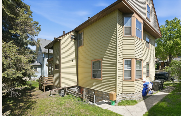
Rear stairwell to basement unit
