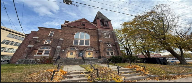
Exterior — Brick Facade
