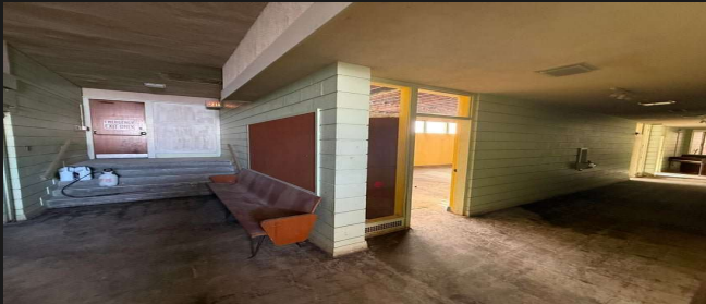
Lower Level Corridor
