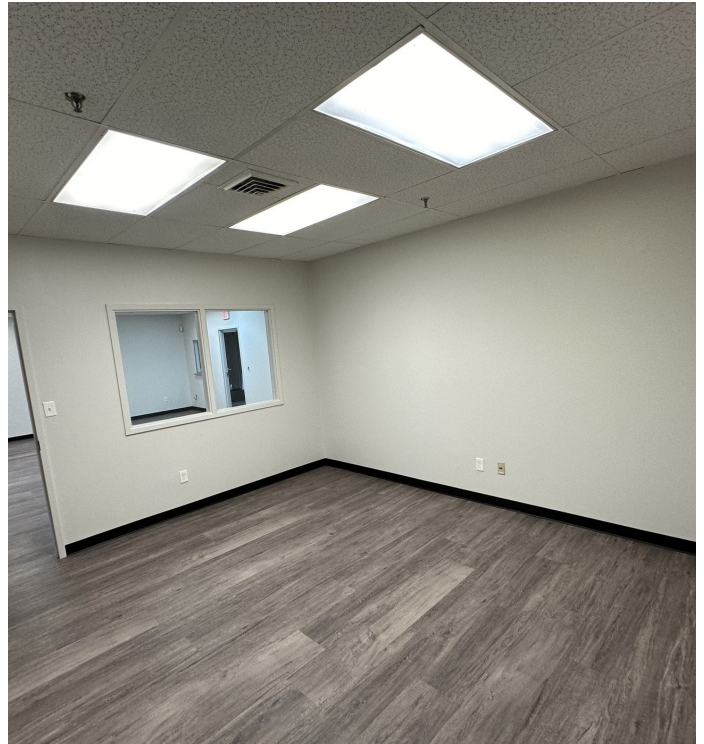
Renovated Office with New Paint + LVT
