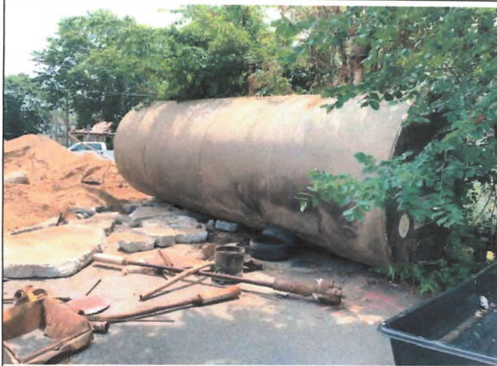
Photograph No. 5: Gasoline tank staged on asphalt following removal
