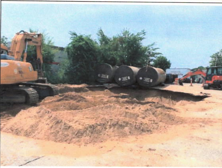
Photograph No. 14: Three gasoline USTs staged on asphalt, excavation partially backfilled
