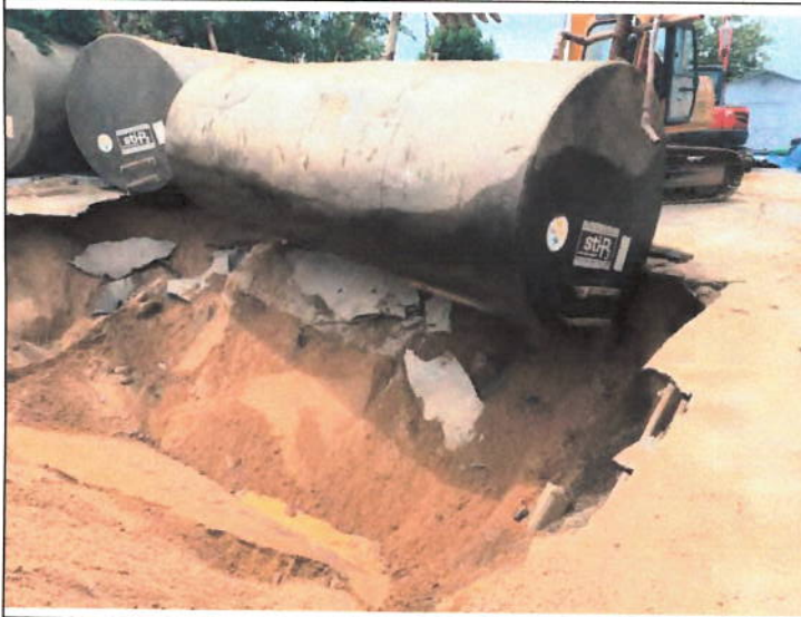
UST Closure 621 Boston Post Road Old Saybrook, CT
