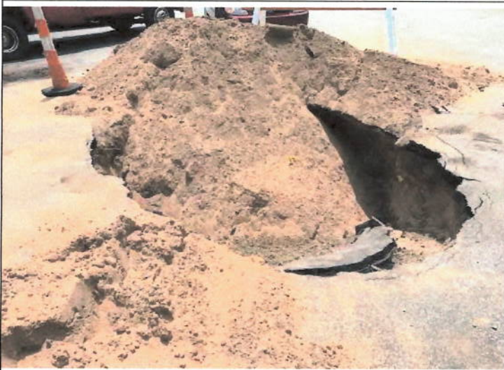
Photograph No. 6: Heating oil tank grave partially backfilled prior to sampling
