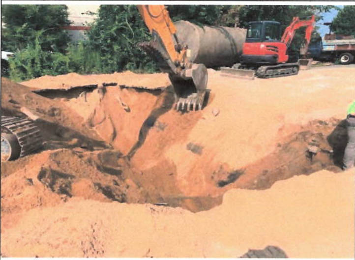
Photograph No. 9: Exposing second gasoline tank at start of second day
