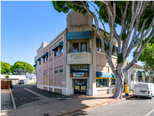
Marsh Street — Building Facade
