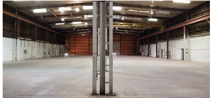
5 TON AND 10 TON CRANES SERVED BY INTERIOR LOADING DOCK
