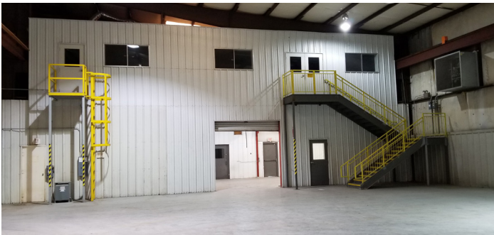
MEZZANINE OFFICE WITH CLIMATE CONTROLLED AREA BELOW
