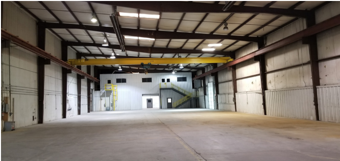
EAST BAY - 5 TON CRANE BAY WITH MEZZANINE OFFICE AT REAR
