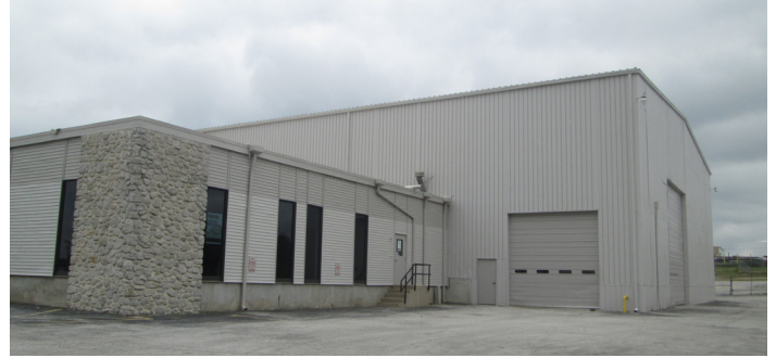
DRIVE THRU BAY (WEST/EAST) WITH INTERIOR DOCK (SOUTH DOOR)
