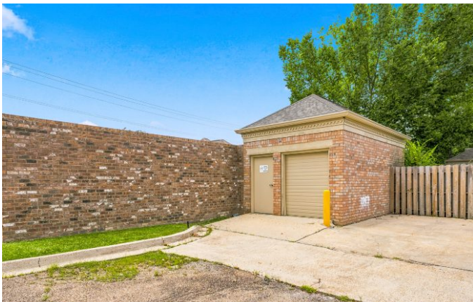
The maintenance building, with a roll-up door beside the screened service wall. The oxygen system serving the building sits behind that wall, not inside the maintenance building.
