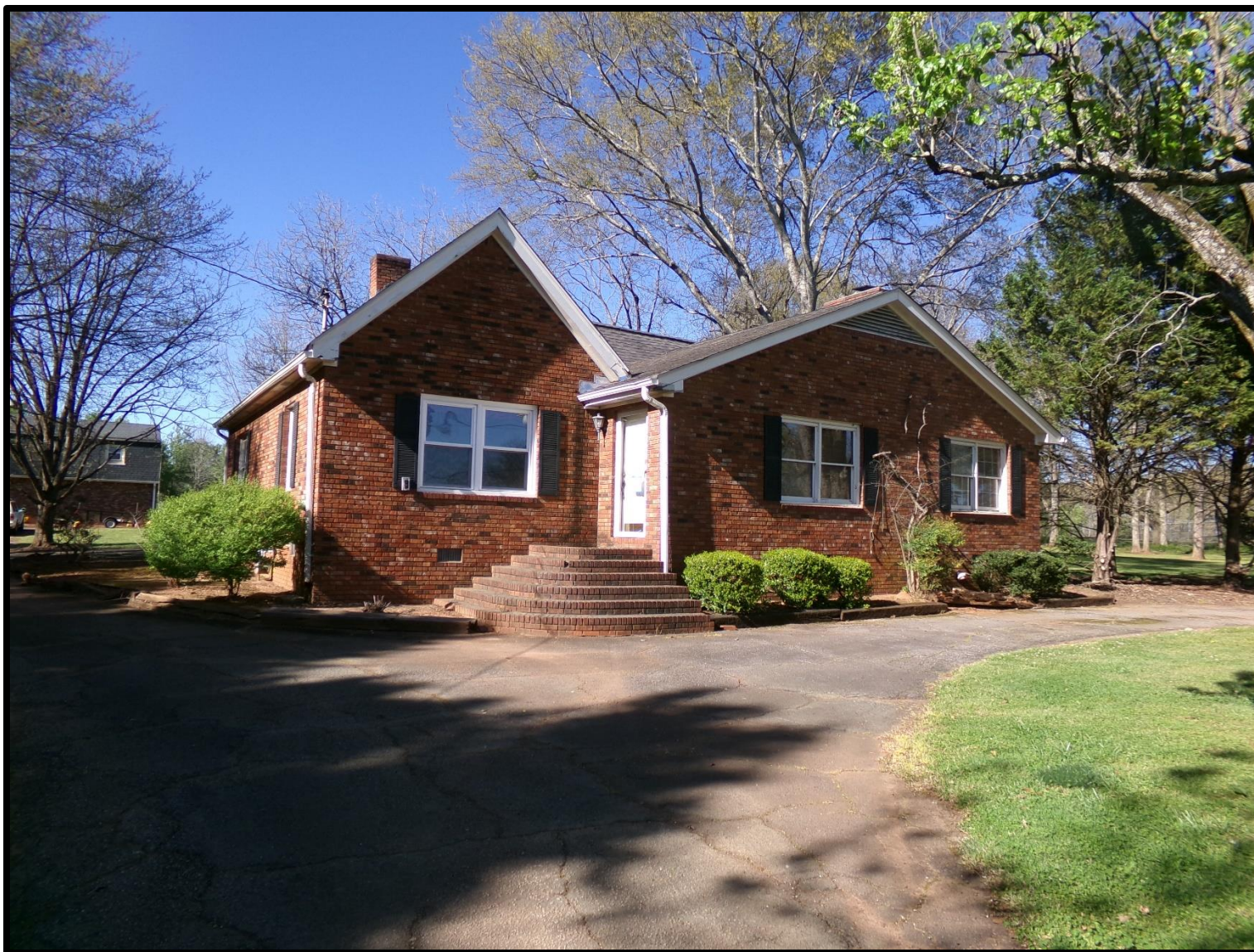
PHOTO 20 - FRONT VIEW OF DWELLING
