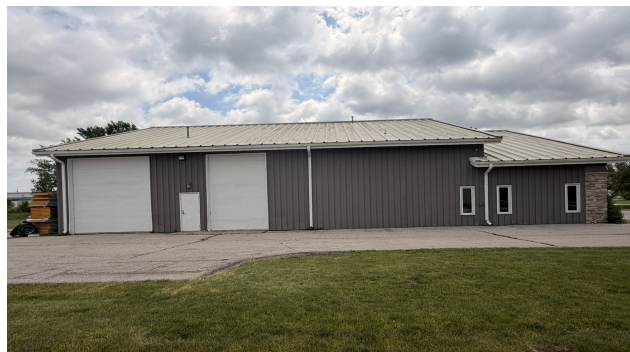
EXTERIOR - OVERHEAD DOORS
