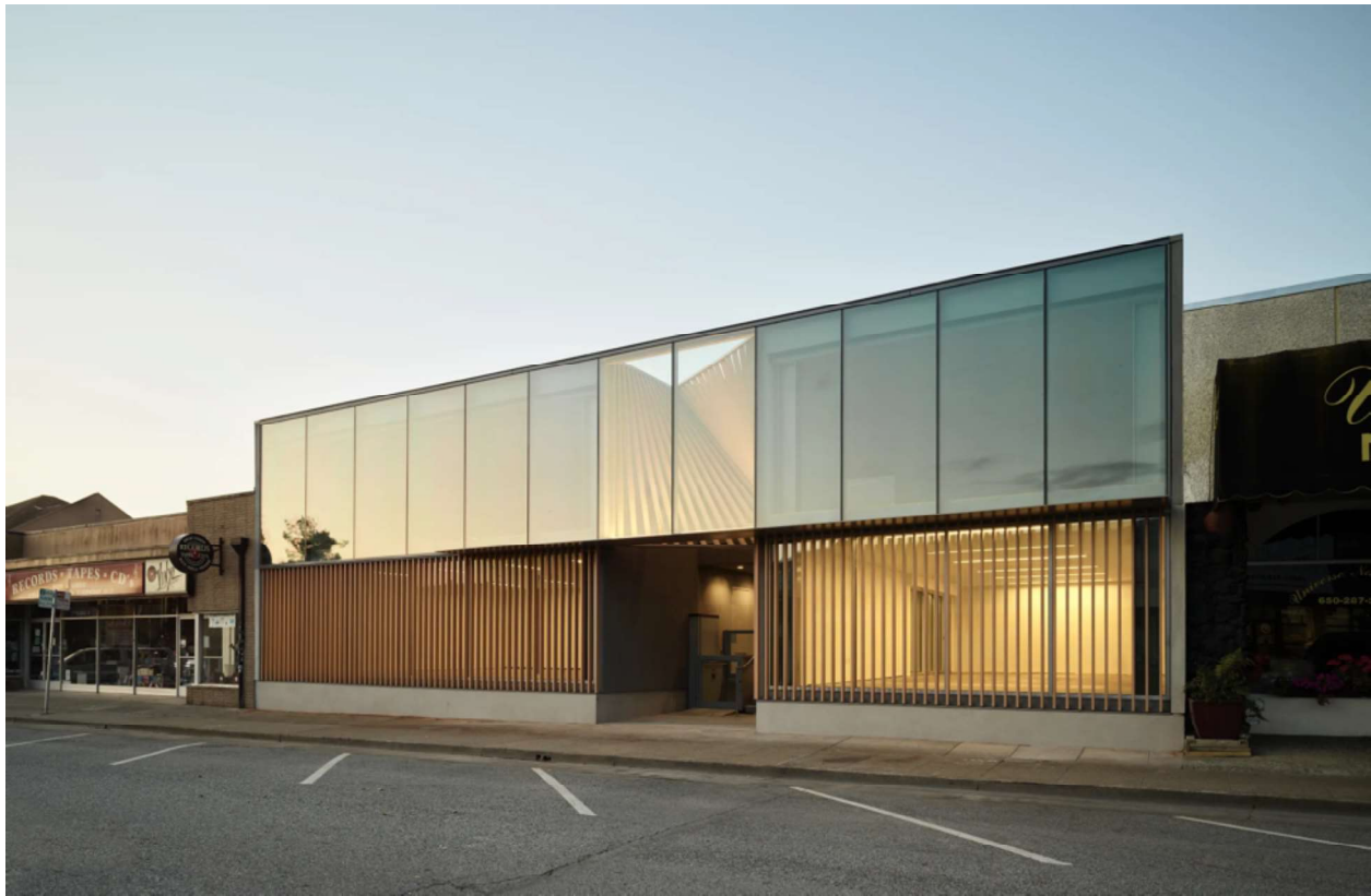
A vertical wood screen shields the ground-level offices from the sun while providing privacy. Photo © Matthew Millman
