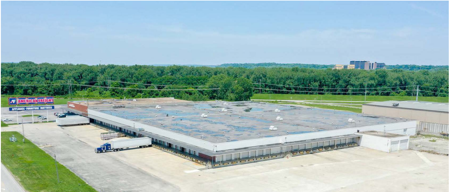
3630 E. Front Street | Kansas City, MO 246,000 +/- square feet
