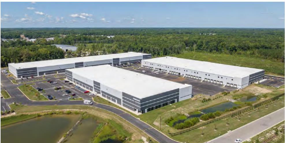
Northlake II 5-Building, 655,000 SF Industrial Park
