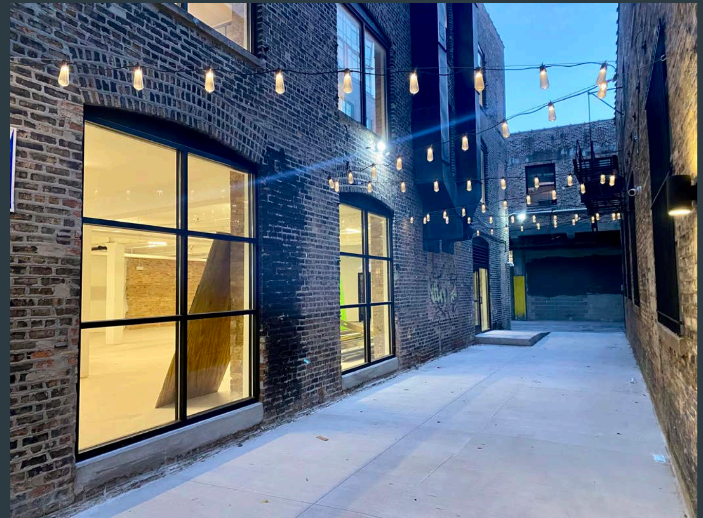
WINDOWS ALONG ALLEYWAY PATIO
