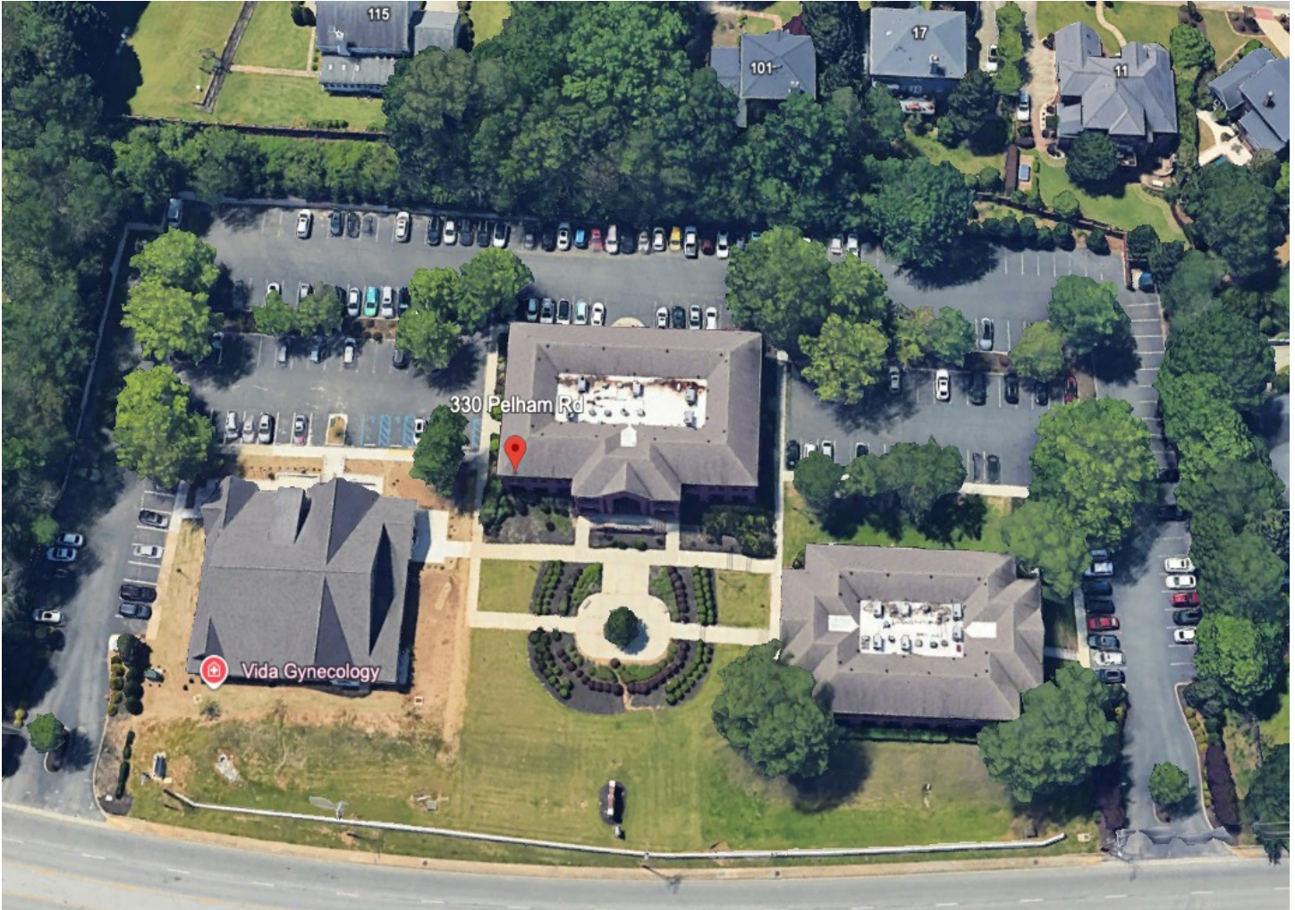
330 Pelham Road campus — Building 100 (pinned) with adjacent office and medical buildings, central courtyard, and wrap-around surface parking fronting Pelham Road.
