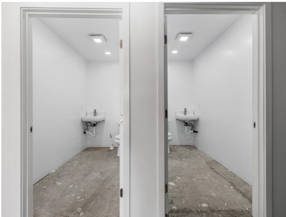
Bathrooms Off of Hallway
