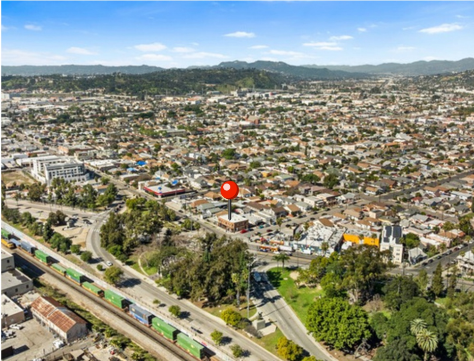
View Facing North
