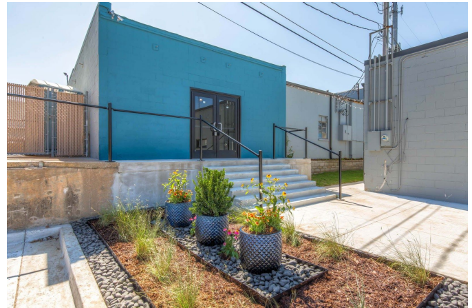
FC TULSA NE Entrance to FCZ Building
