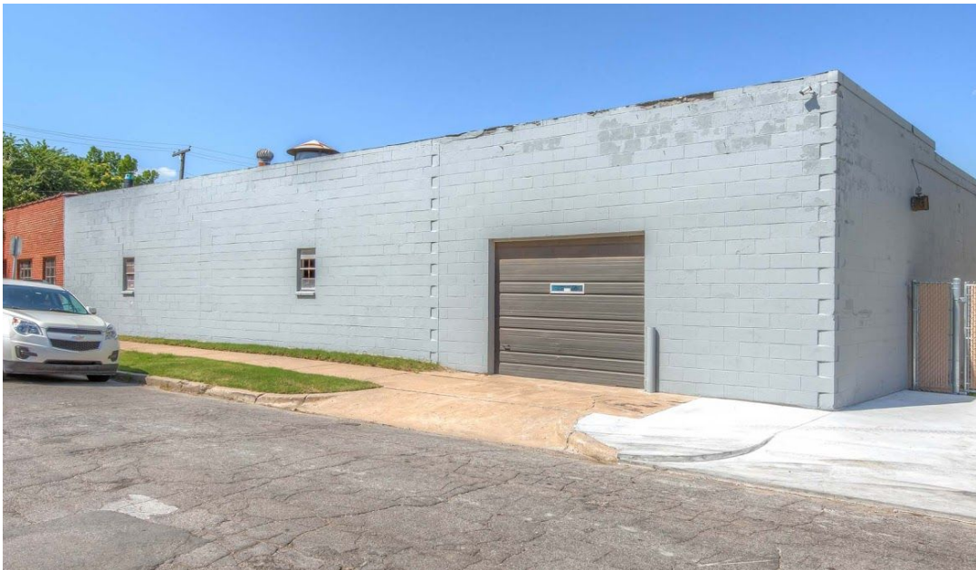
NE Entrance - FCZ Building - Current
