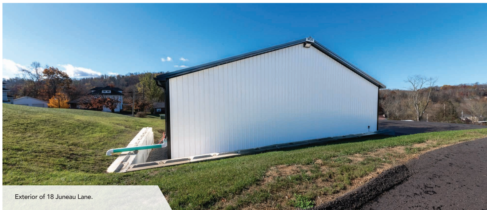
Exterior of 18 Juneau Lane.
