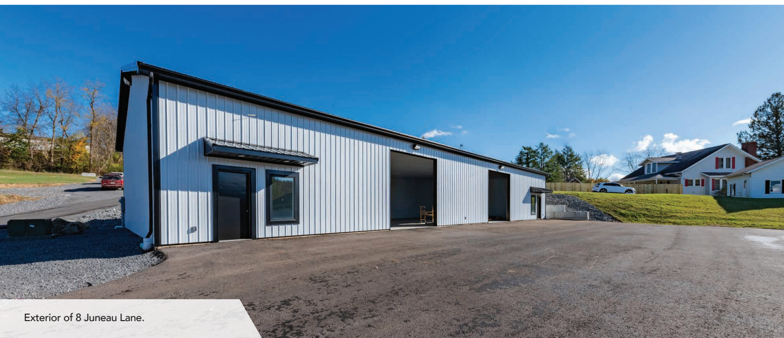
Exterior of 8 Juneau Lane.
