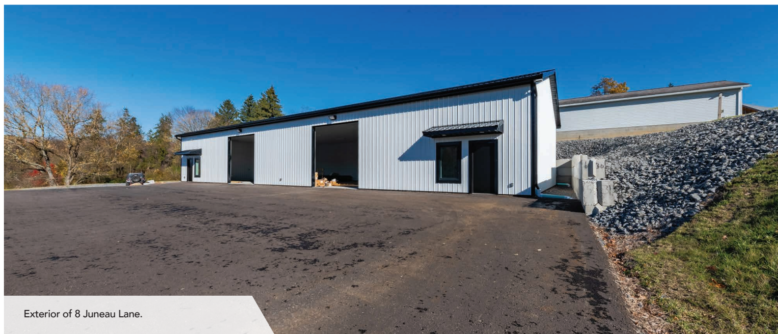
Exterior of 8 Juneau Lane.
