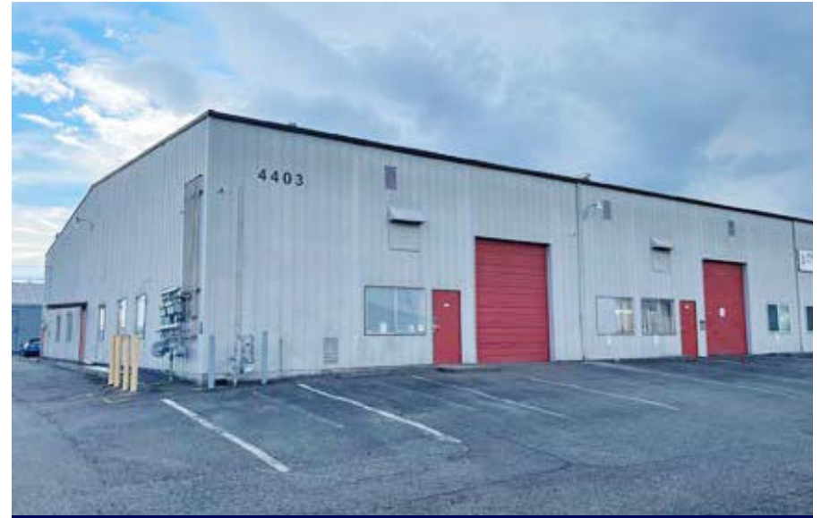
4403 Russell Road Building
