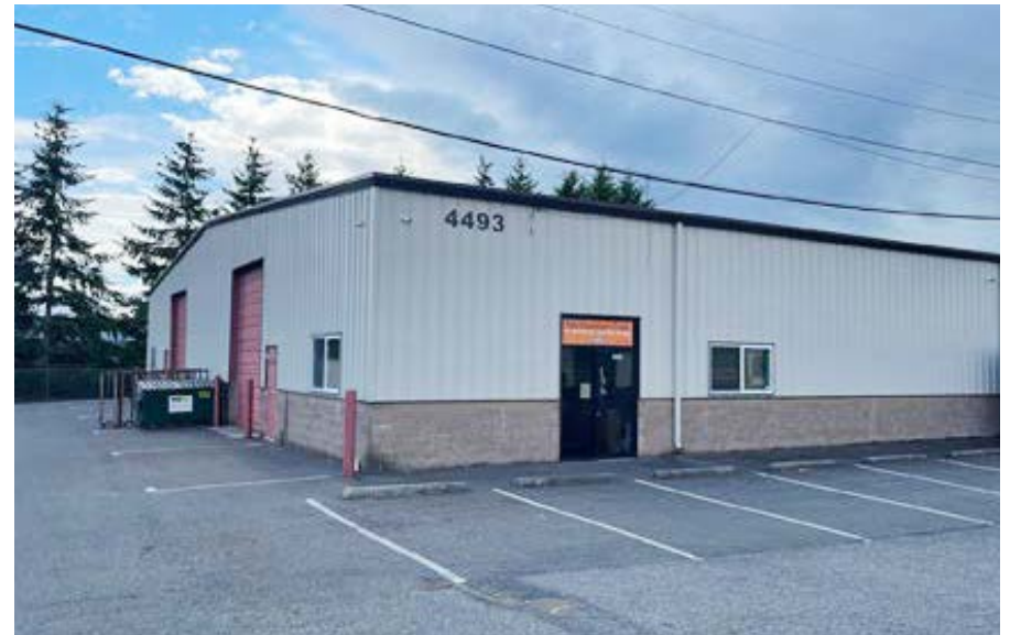
4493 Russell Road Building
