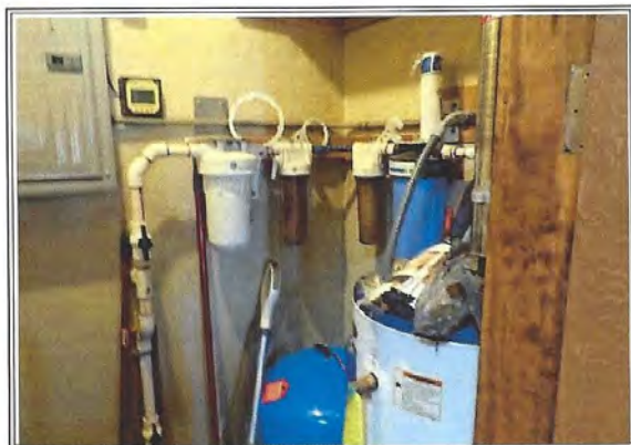
HOT WATER HEATER AND WATER FILTER SYSTEM
