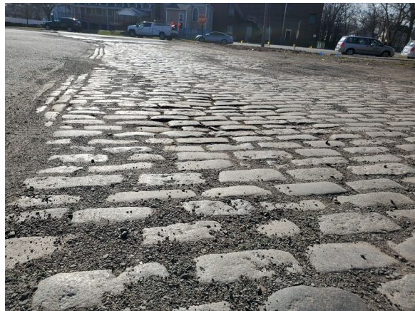
Photo 8 - Cobblestone surface of Laurel Street
