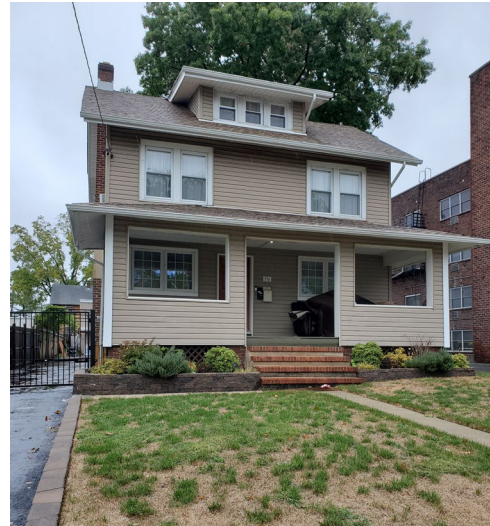
Photo 1 – Dwelling on Block 3802, Lot 25
